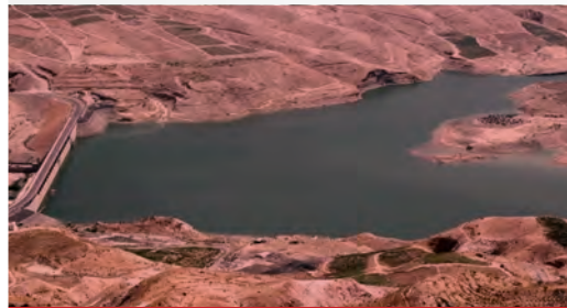
Electrical Energy Storage Project near Wadi Al-Mujib Dam
